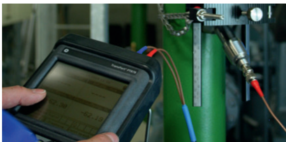
Figure 4: One of the ultrasonic probes, which transmits the flow-through data to the mobile measuring device.
