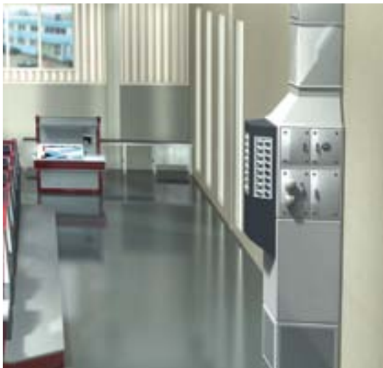
Air for removal of heat from printing press. Circulating air for reduction of dust and heat recovery
